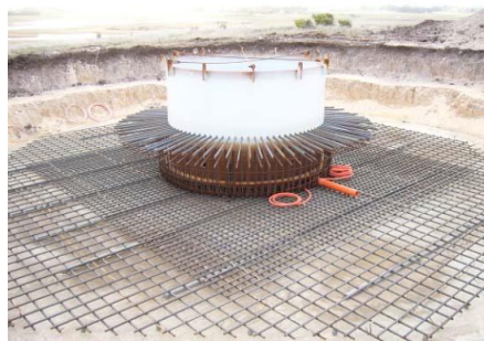
Plate 2-2 Steel reinforcement being added
