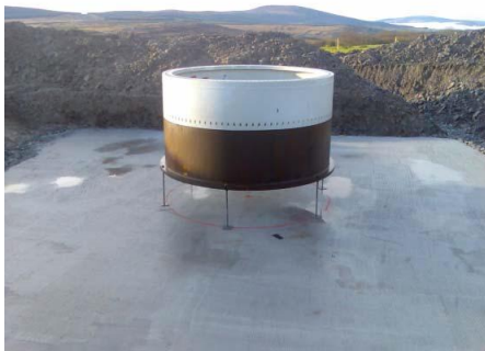
Plate 2-1 Levelled turbine tower “can”
